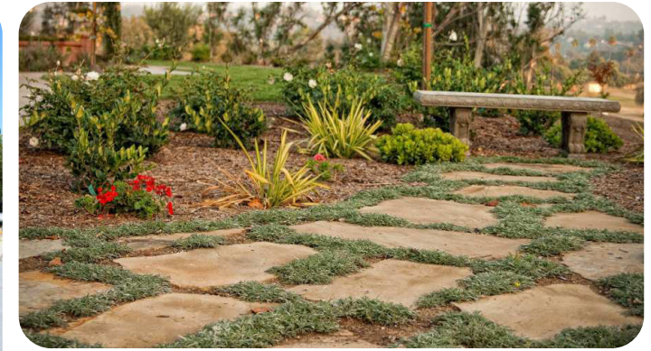
STEPPERS WITH GROUNDCOVER NOT TO EXCEED 3' X 3' IN SIZE SPACED AT LEAST 2" APA
