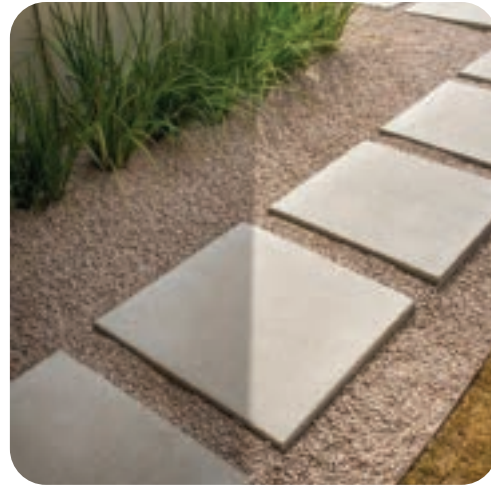
CONCRETE STEPPERS / PATHWAY NOT TO EXCEED 3' X 3' IN SIZE SPACED AT LEAST 2" APART
