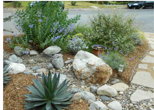
SUSTAINABLE FEATURE: A dry river bed is an area designed to slow heavy flows of water from rainfall and correct erosion problems. It is made up of a shallow swale lined with stone large enough to slow the speed of storm water and prevent erosion.
