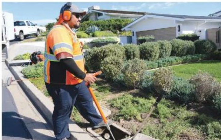
MWDOC leak detection technicians use listening equipment to find hidden leaks.
