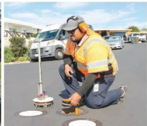
MWDOC leak detection technicians use listening equipment to find hidden leaks.
