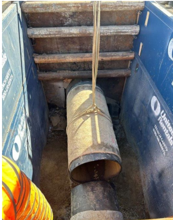
OC Feeder Shutdown - Access Point for Liner Replacement
