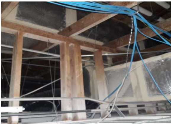
Ducts above the ceiling with foil backed insulation
