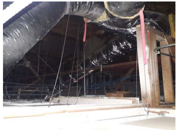
Above Ceiling, Fiberglass insulated ducts
