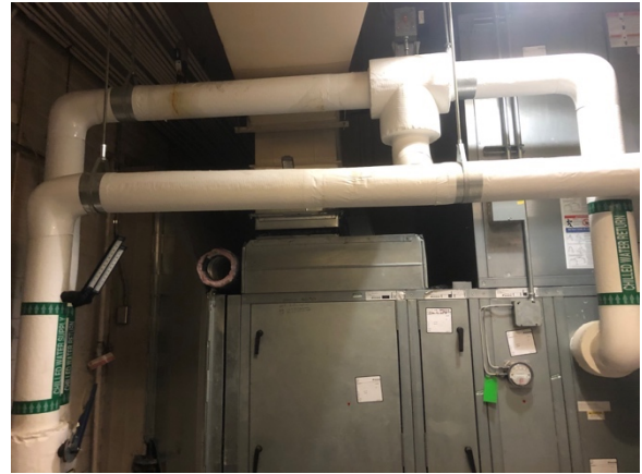
Typical Fiberglass Insulation
