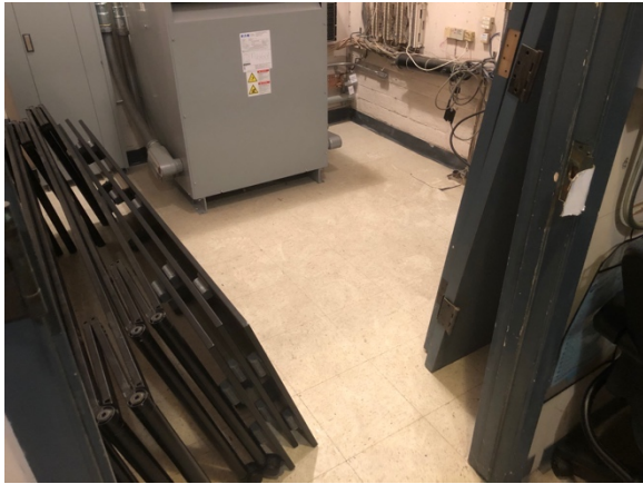
Tile and Mastic are ACM in the Electrical Room
