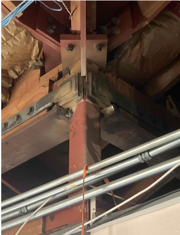
Structural Reinforcement to Southwest Interior Corner of Building
