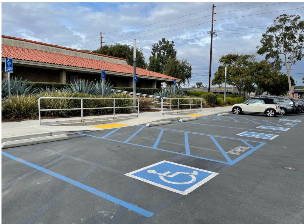
Restriped ADA Parking Spaces and Upgraded Truncated Domes to meet ADA Requirements
