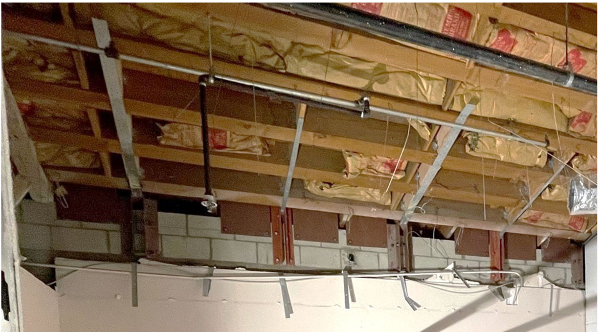
Wood Reinforcement and Strapping in the Southeast Corner of the Building
