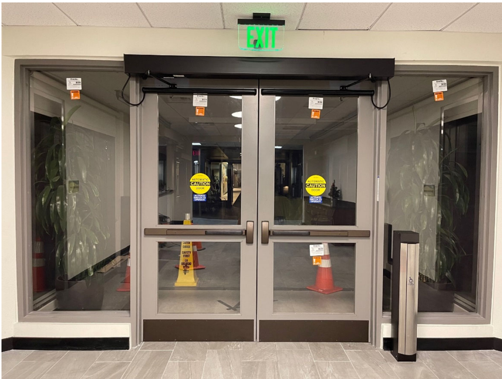
New ADA/Fire Code Compliant Lobby Doors (MWDOC Side)
