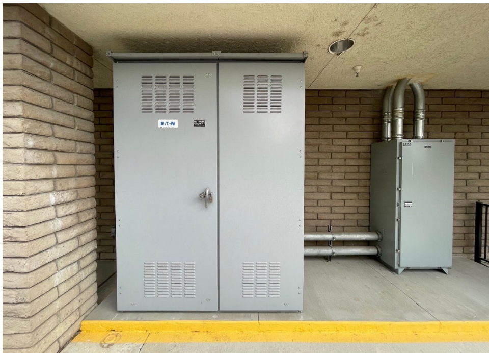
Upgraded Main Switchboard for the MWDOC Building
