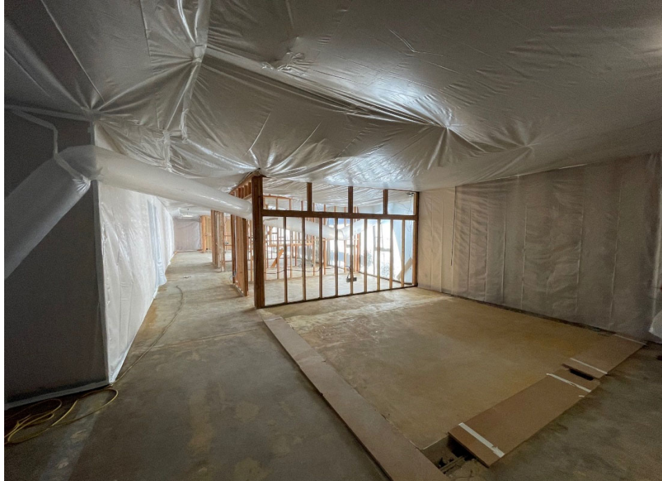
Asbestos Mitigation and Monitoring During Demolition
