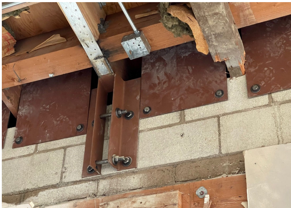
Bent Plates and Structural Brackets Attached to Interior Wall
