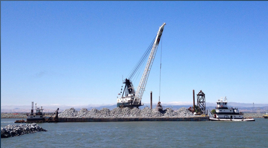
Emergency Drought Barrier Installation in 2015
