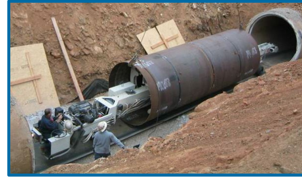
Pipeline Relining $493 million
