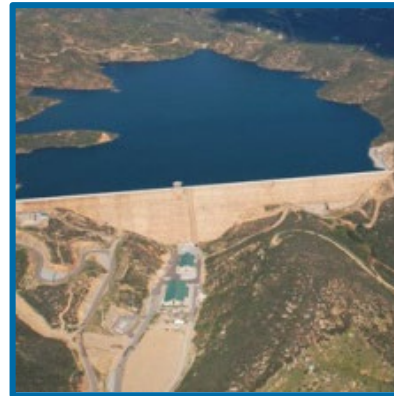
Olivenhain Dam & Reservoir $198 million
