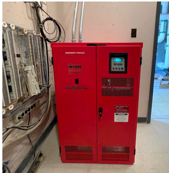
Emergency Lighting Batteries
