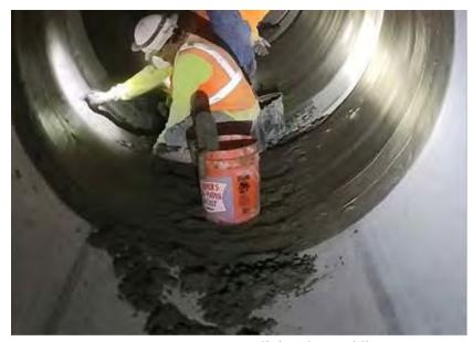
Contractor cement mortar lining the steel liner
