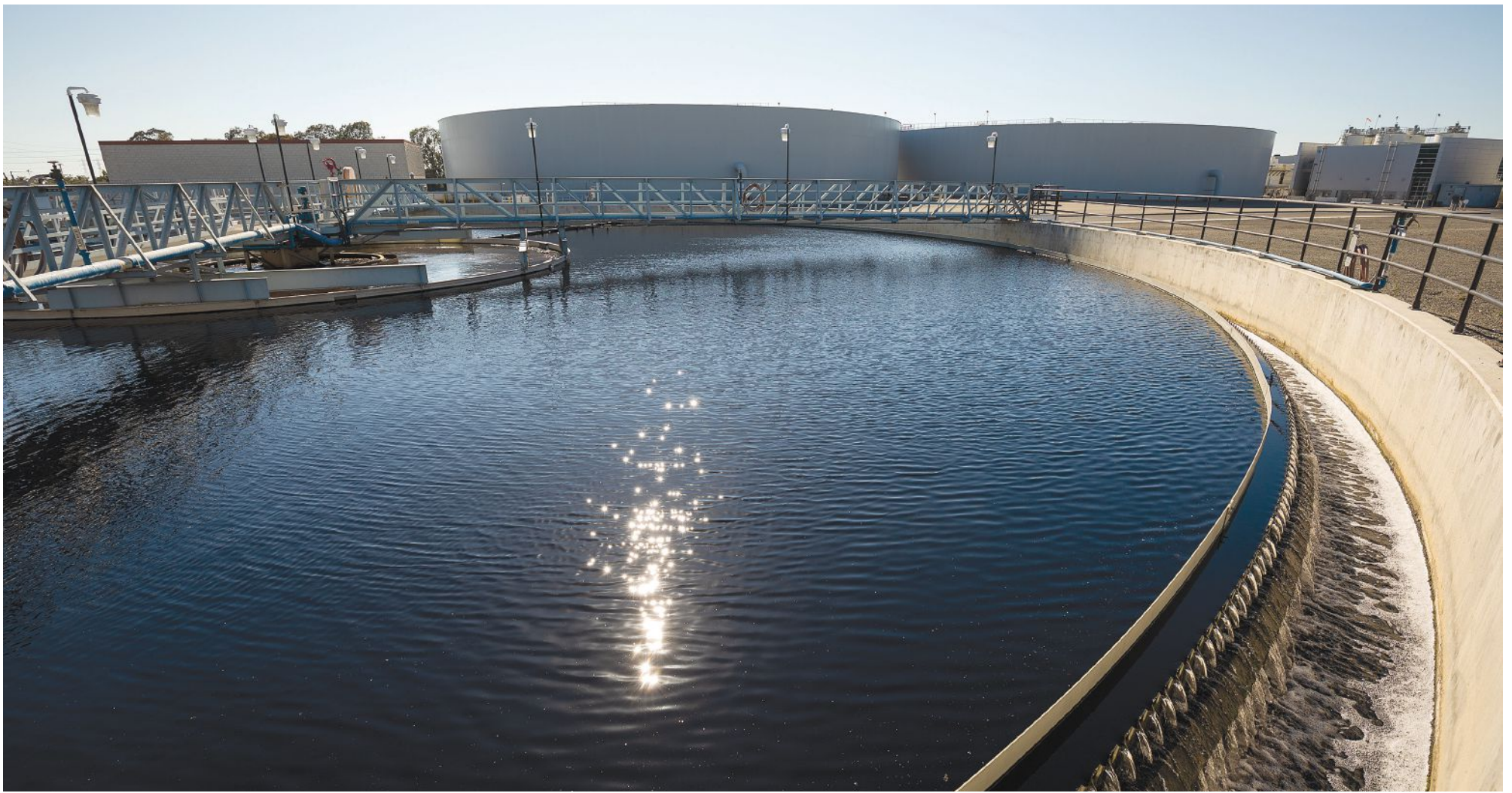
Secondary clarifiers are part of the wastewater treatment process removing organic materials that were not removed through primary treatment. Treated water is then sent to the Groundwater Replenishment System for recycling or is released into the ocean.
