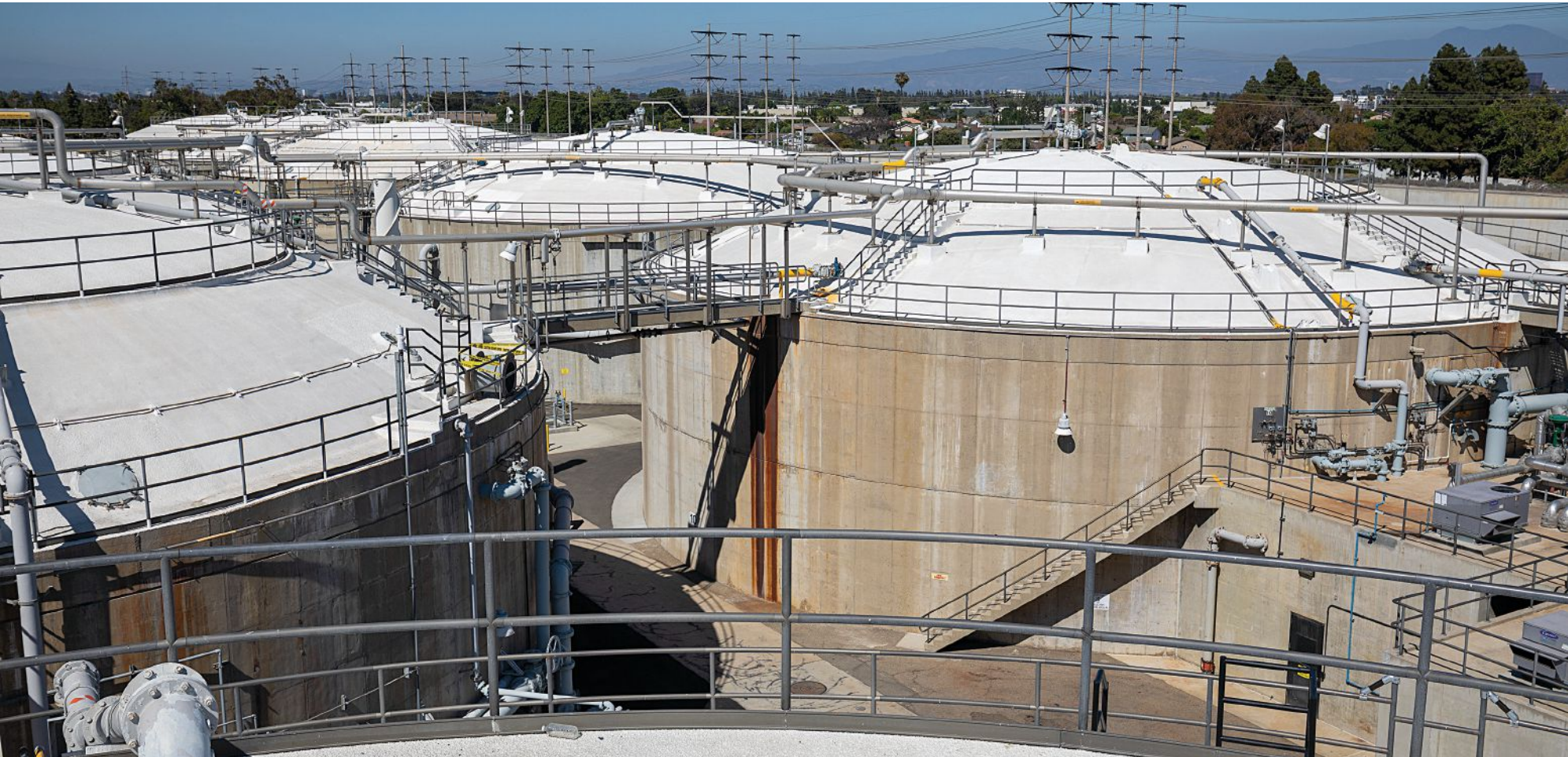
Solids captured from the treatment process are loaded into anaerobic digesters where they are heated to about 98 degrees and treated for 18-21 days. The digestion process produces methane gas and a material called biosolids which are composted and used as a soil amendment.
