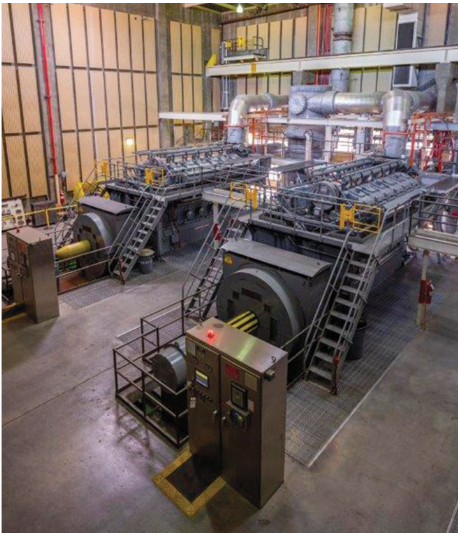
The Central Power Generation System has eight clean burning, internal combustion engines that power generators producing more than 60 percent of the power required to run our two treatment plants in Huntington Beach and Fountain Valley. This system is fueled by renewable methane generated in OCSD’s anaerobic digesters.
