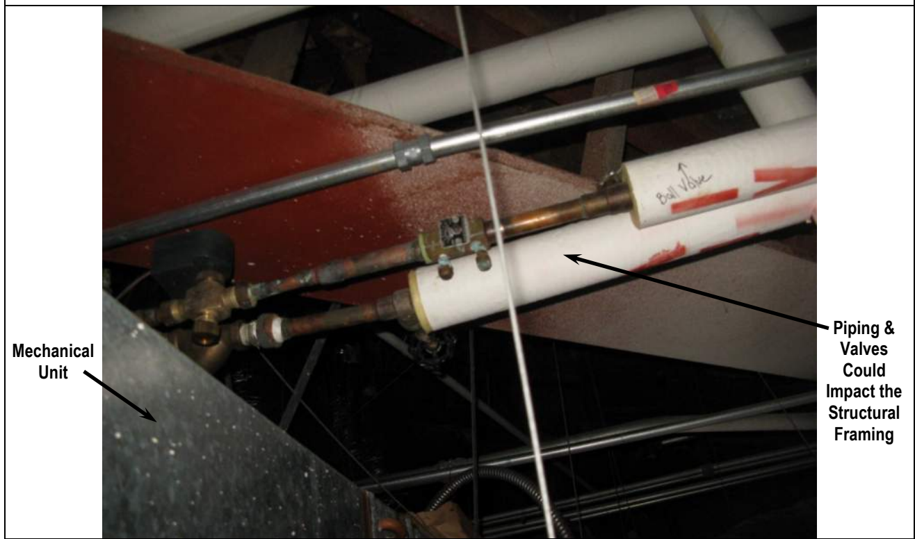
Photo 26: Water Piping in Ceiling Above Computer Room
