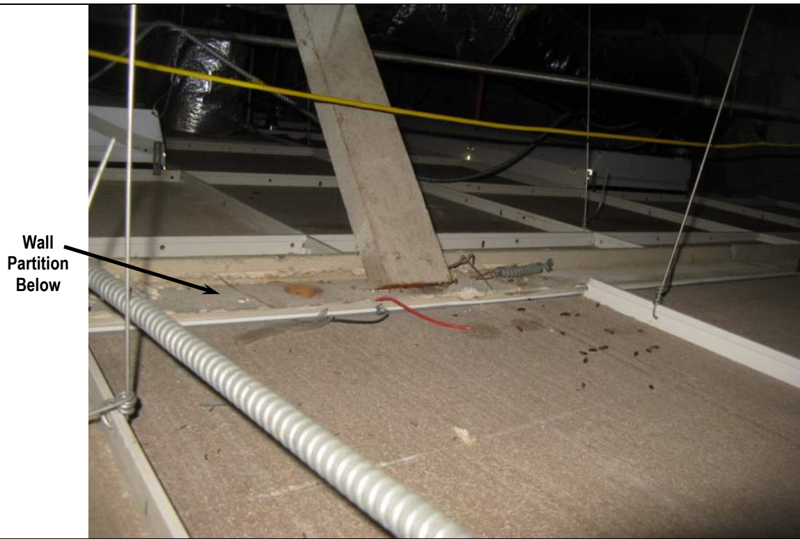
Photo 16: Widely Spaced, Steeply Sloped and Inadequate Brace Connection
