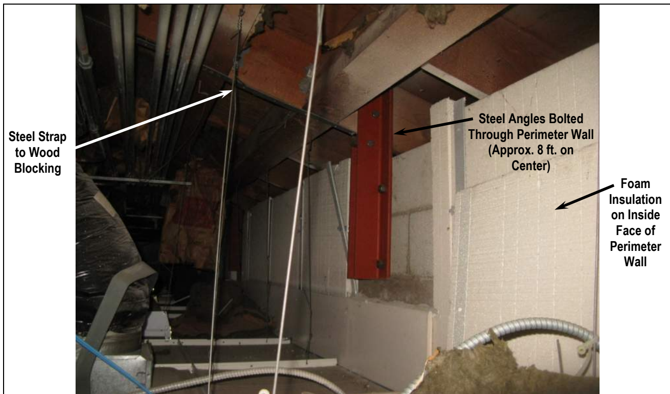
Photo 9: Typical Out of Plane Wall Anchorage Connection
