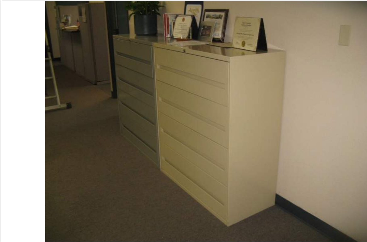
Photo 22: Unanchored Tall Narrow Contents in Hallway
