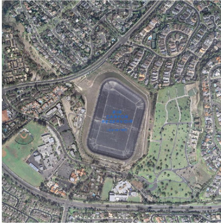
Figure 7-17: View of Big Canyon Dam and Reservoir (North to the top; photo courtesy of City of Newport Beach; December 2007)
