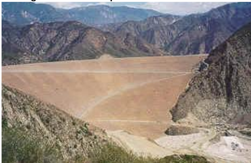
Figure 7-15: View Upstream of Seven Oaks Dam
