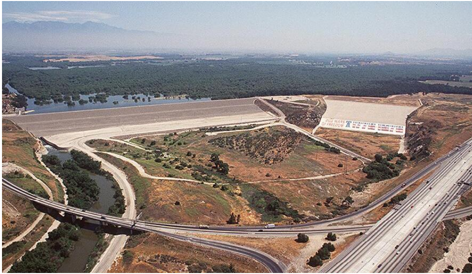
Figure 7-14: View to the North of Prado Dam (to the right-center), and Prado Dam Reservoir (in the Background)
