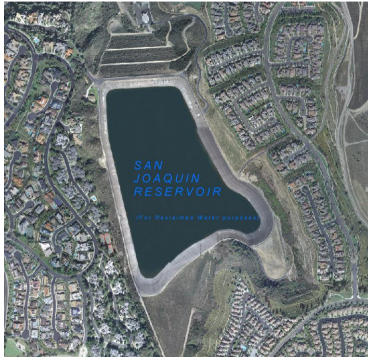
Figure 7-16: View of San Joaquin Dam (at the top) and Reservoir (North is to the top; photo courtesy of the City of Newport Beach; December 2007)
