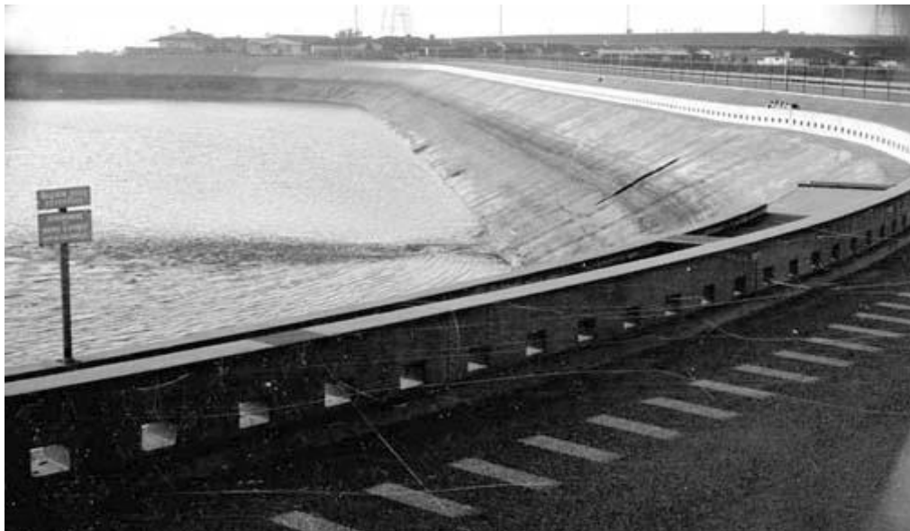
Figure 7-9: Initial Failure of Baldwin Hills Dam. Dark spot in lower right-hand quadrant shows the beginning of the break in the dam.
