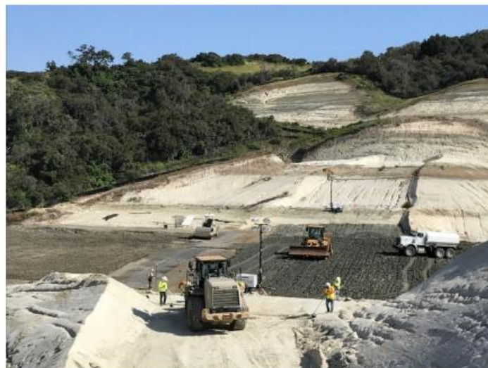
Sukut Compacting Zone 1A Core Material at East Saddle Dam
