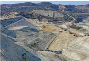
Main Dam: Scrapers Hauling in Embankment Fill
