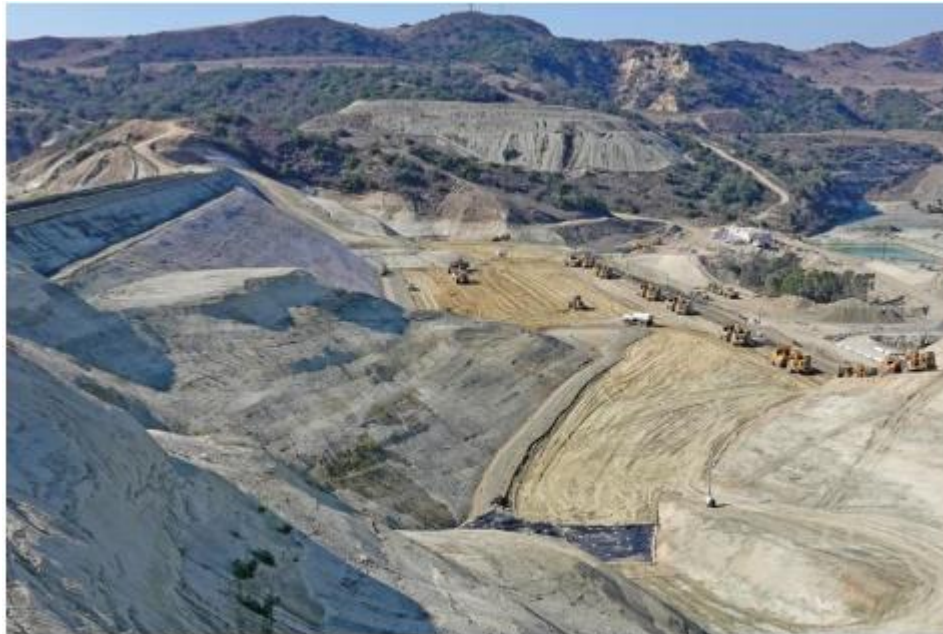
Main Dam: Scrapers Hauling in Embankment Fill
