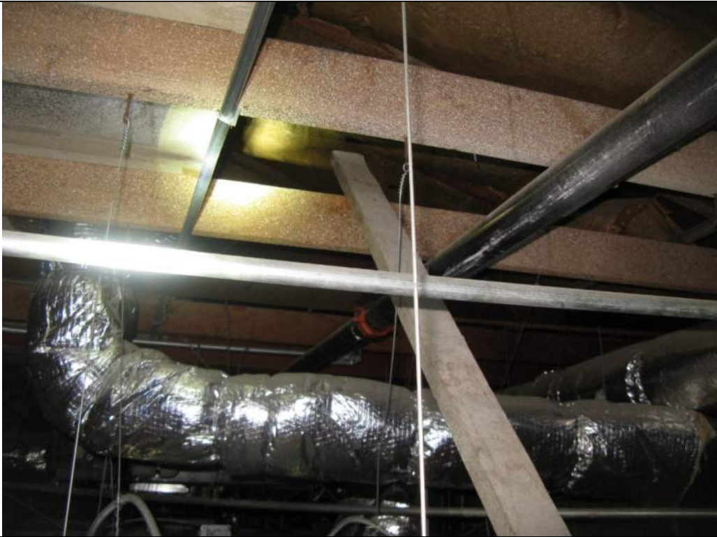
Photo 15: Partition Brace to Unbraced Roof Framing
