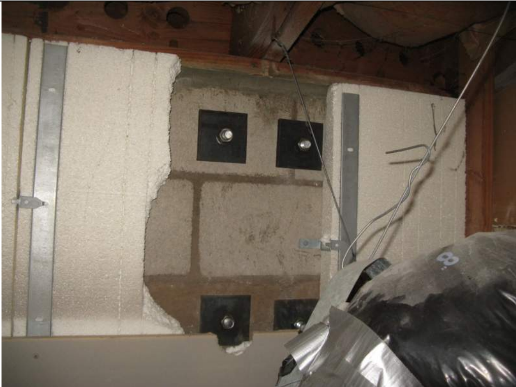
Photo 11: Wall Anchorage Connection Presumed to Exist on Far Side of Wall
