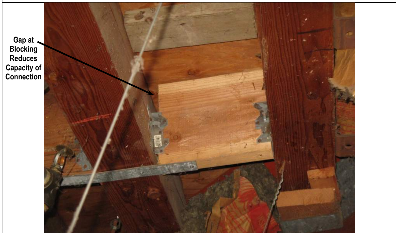
Photo 10: Close-up Showing Gap at Seismic Blocking
