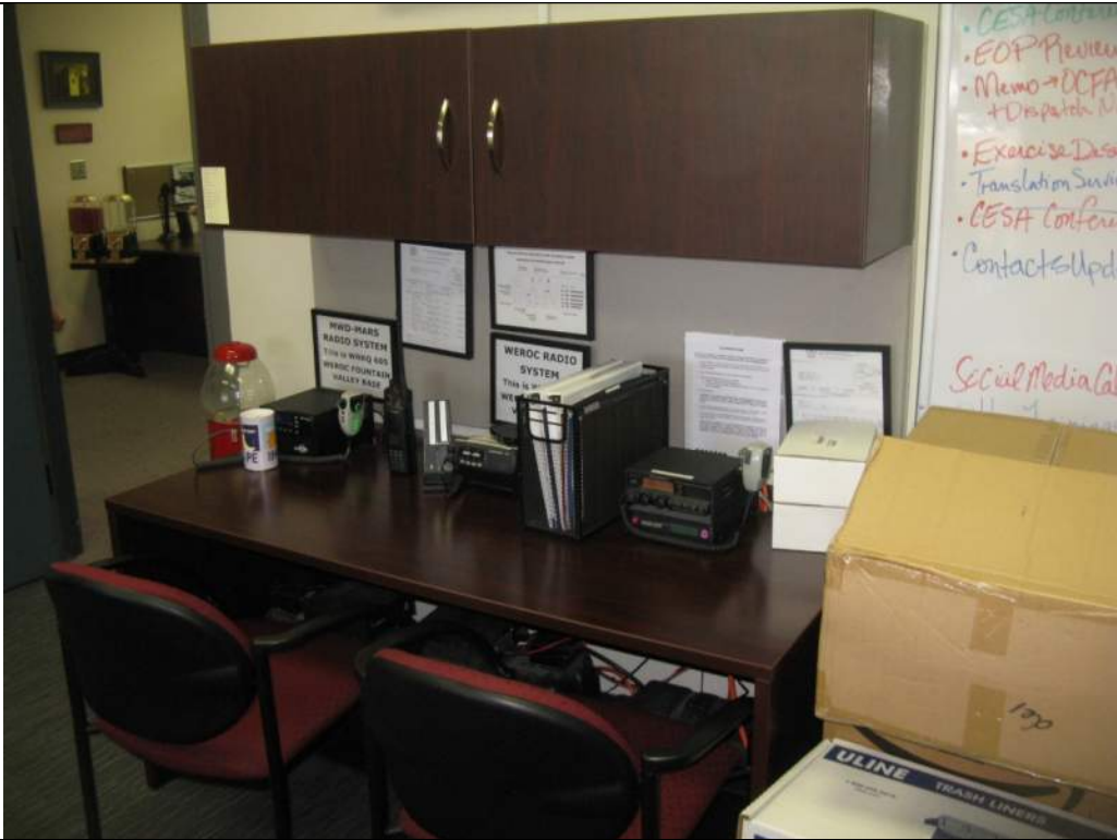
Photo 20: Unrestrained Communications Equipment
