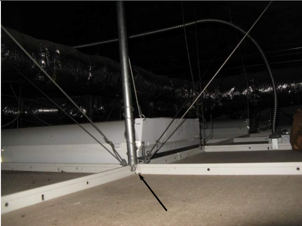
Photo 29: Typical Ceiling Bracing with Compression Post
