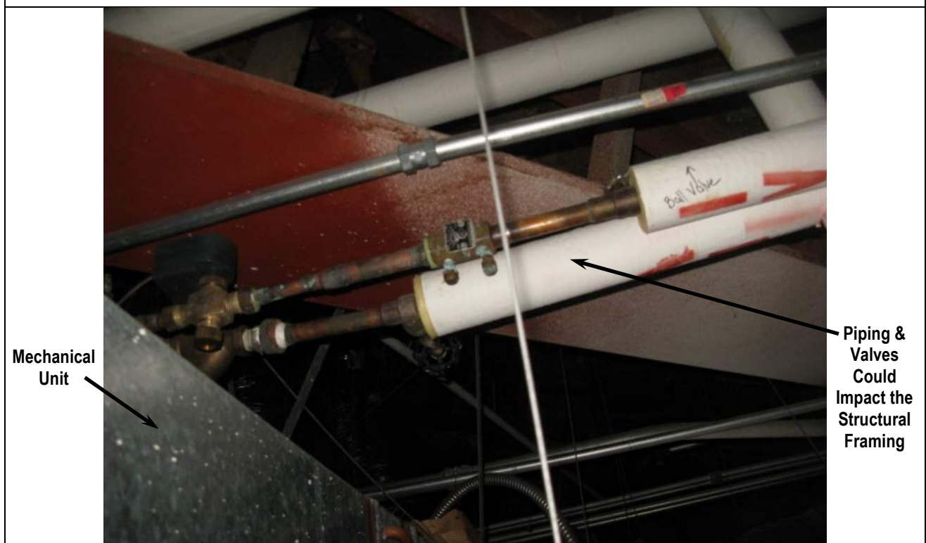
Photo 26: Water Piping in Ceiling Above Computer Room
