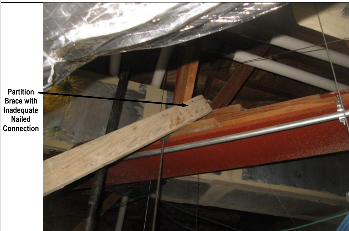
Photo 14: Interior Partition Bracing Connection
