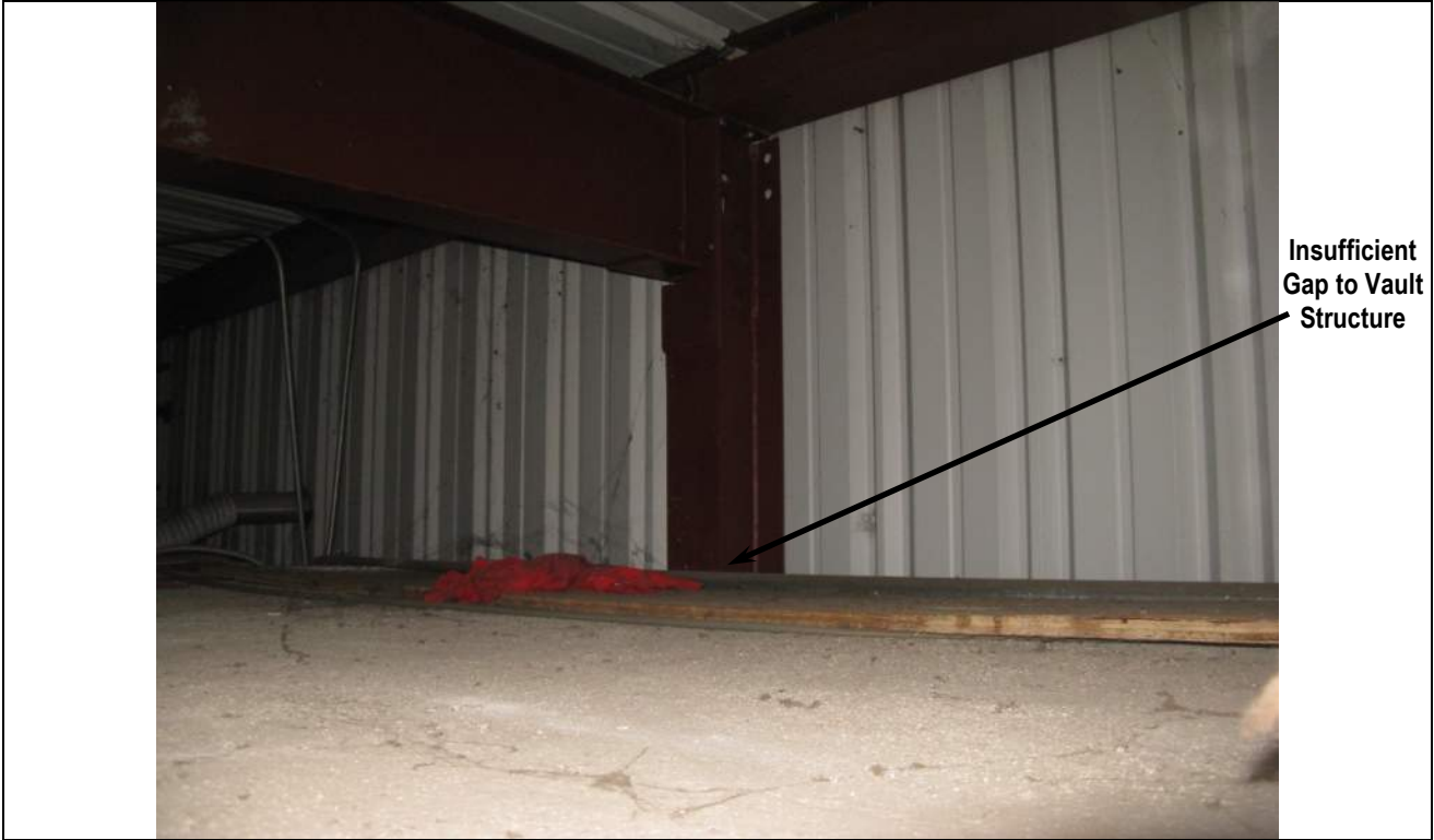
Photo 18: Rigid Frame Abutting Masonry Vault
