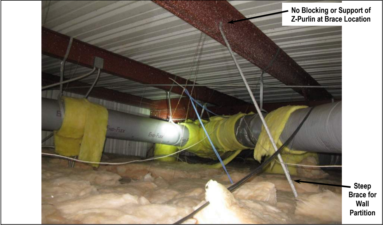
Photo 28: Typical View within Ceiling Space
