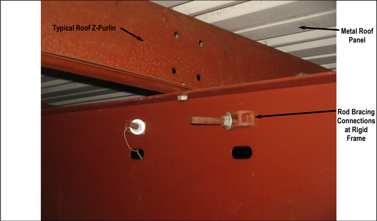
Photo 20: Close-up of Horizontal Rod Bracing Connections
