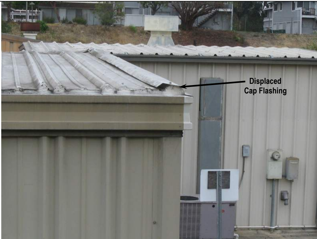
Photo 9: Close-up of Flashing at South End of Roof
