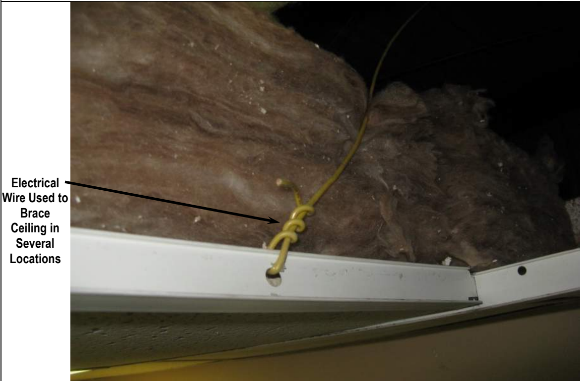
Photo 24: View of Improper Ceiling Support Wire
