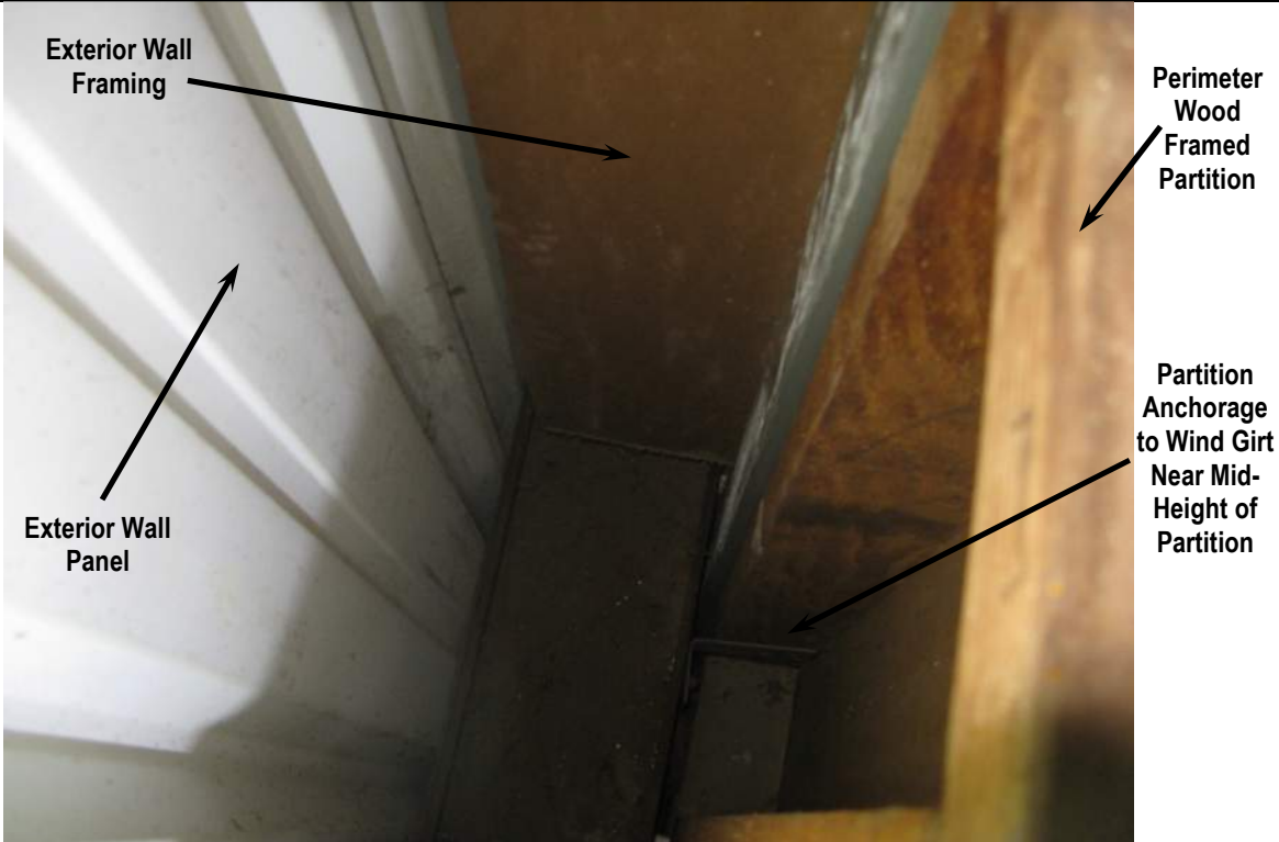
Photo 30: View of Perimeter Partition Attachment (Looking Down)
