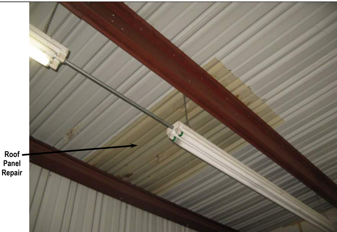
Photo 10: Interior View at Repaired Roof Panel
