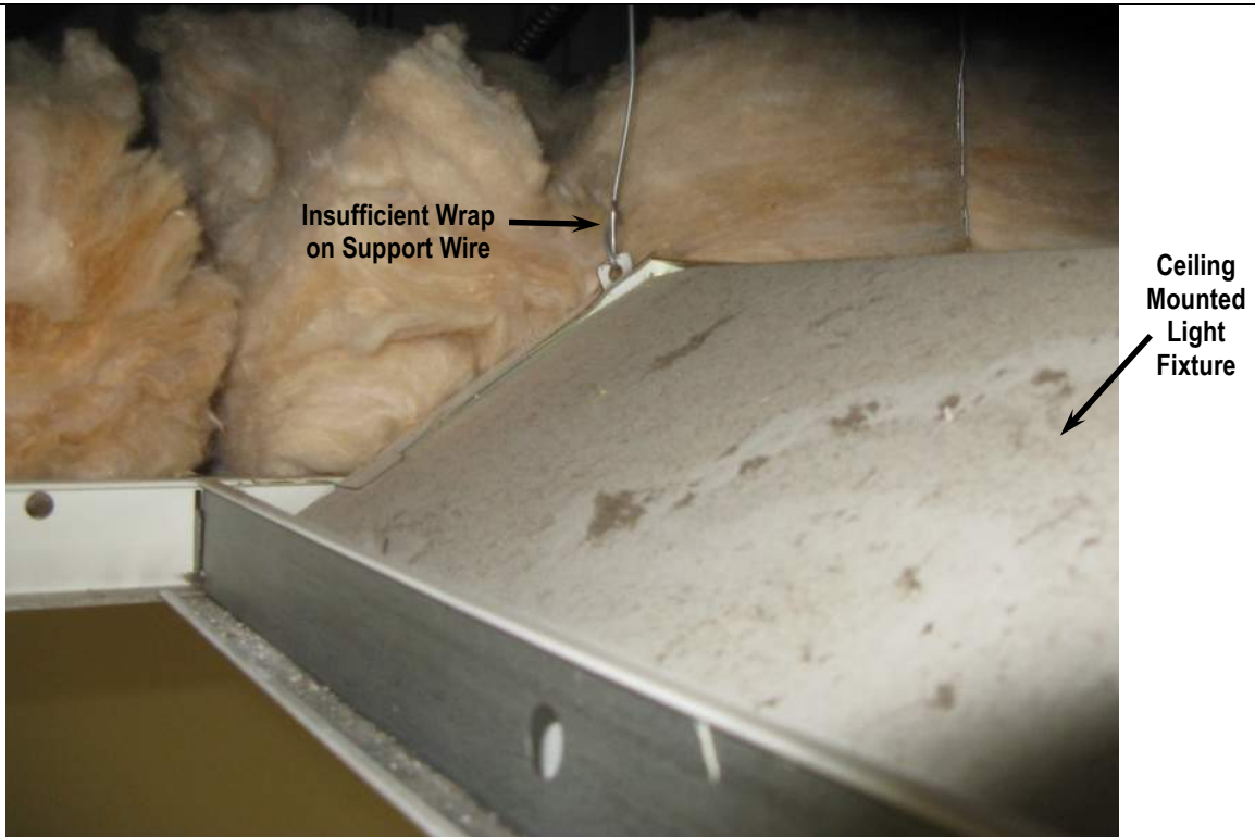
Photo 25: View of Improper Light Support Wire
