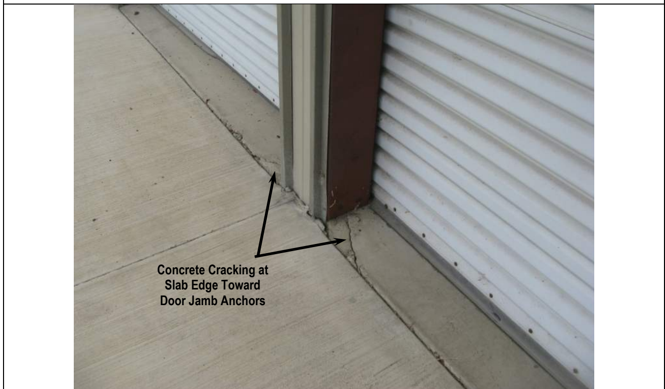
Photo 12: Damaged Concrete at Slab Edge
