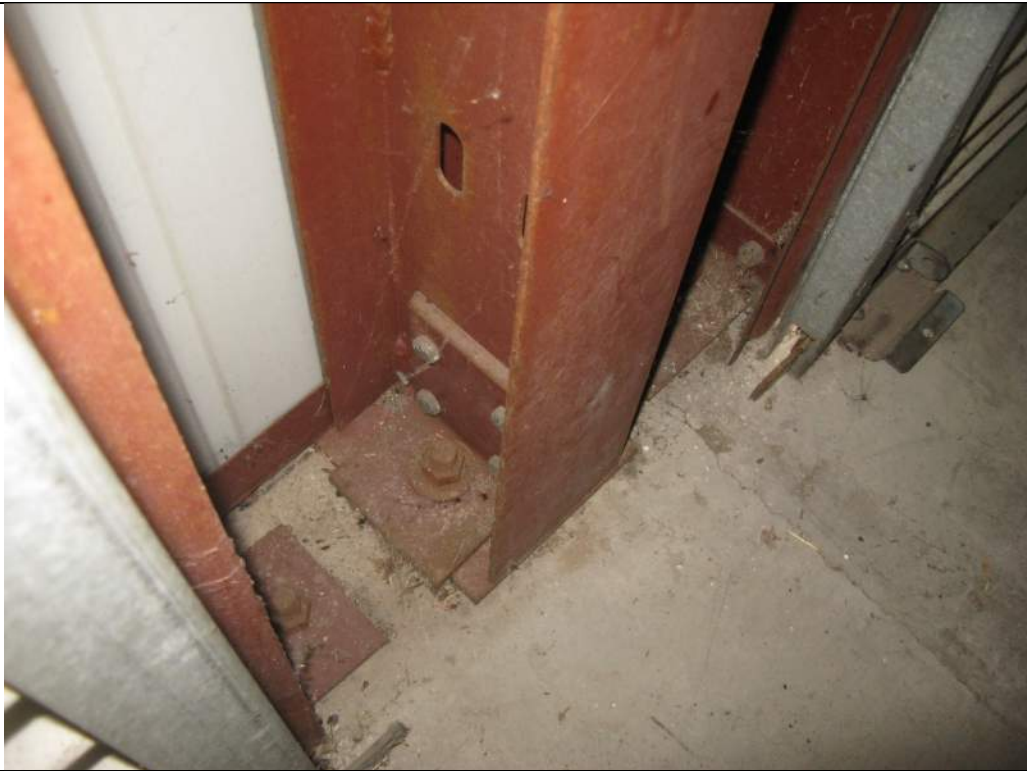
Photo 16: Rigid Frame Base Anchorage in Garage Area
