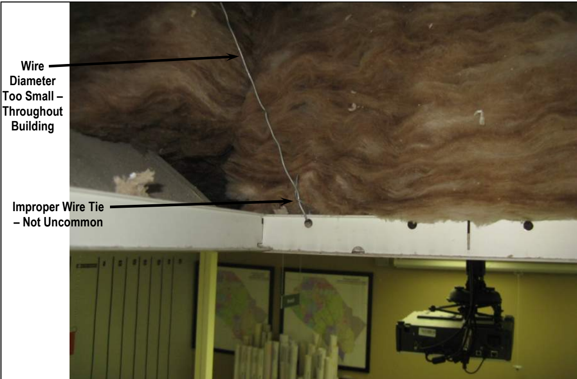
Photo 23: View of Ceiling Support Wire
