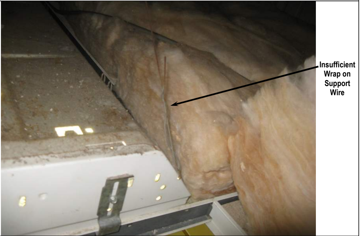
Photo 26: View of Improper Light Support Wire
