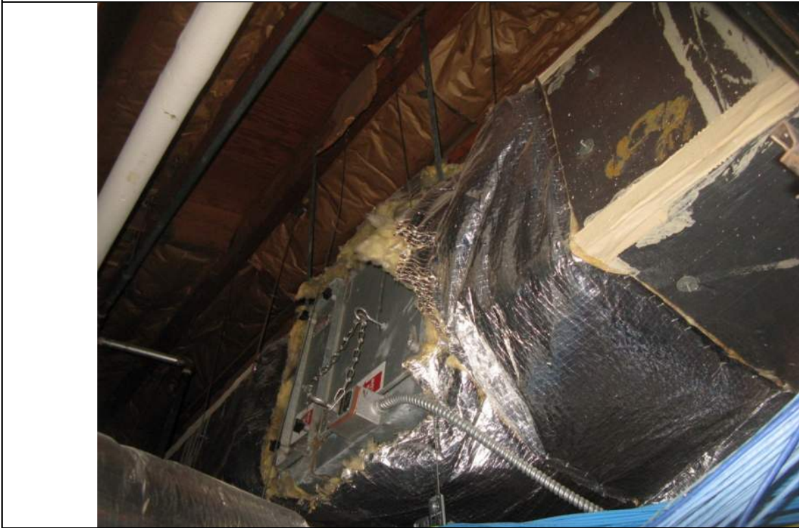
Photo 28: Typical In-Line Mechanical Unit without Seismic Bracing
