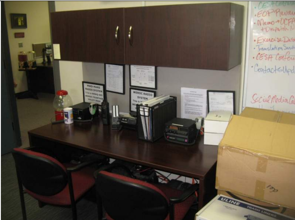
Photo 20: Unrestrained Communications Equipment
