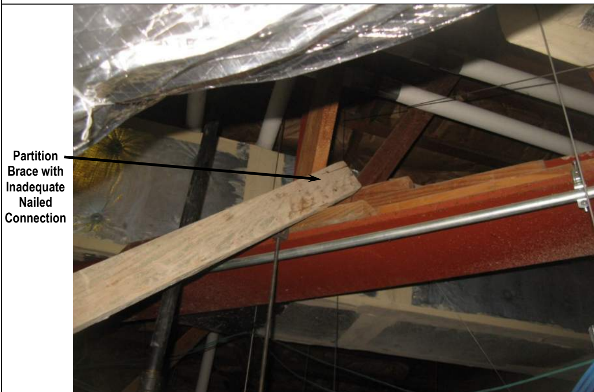
Photo 14: Interior Partition Bracing Connection
