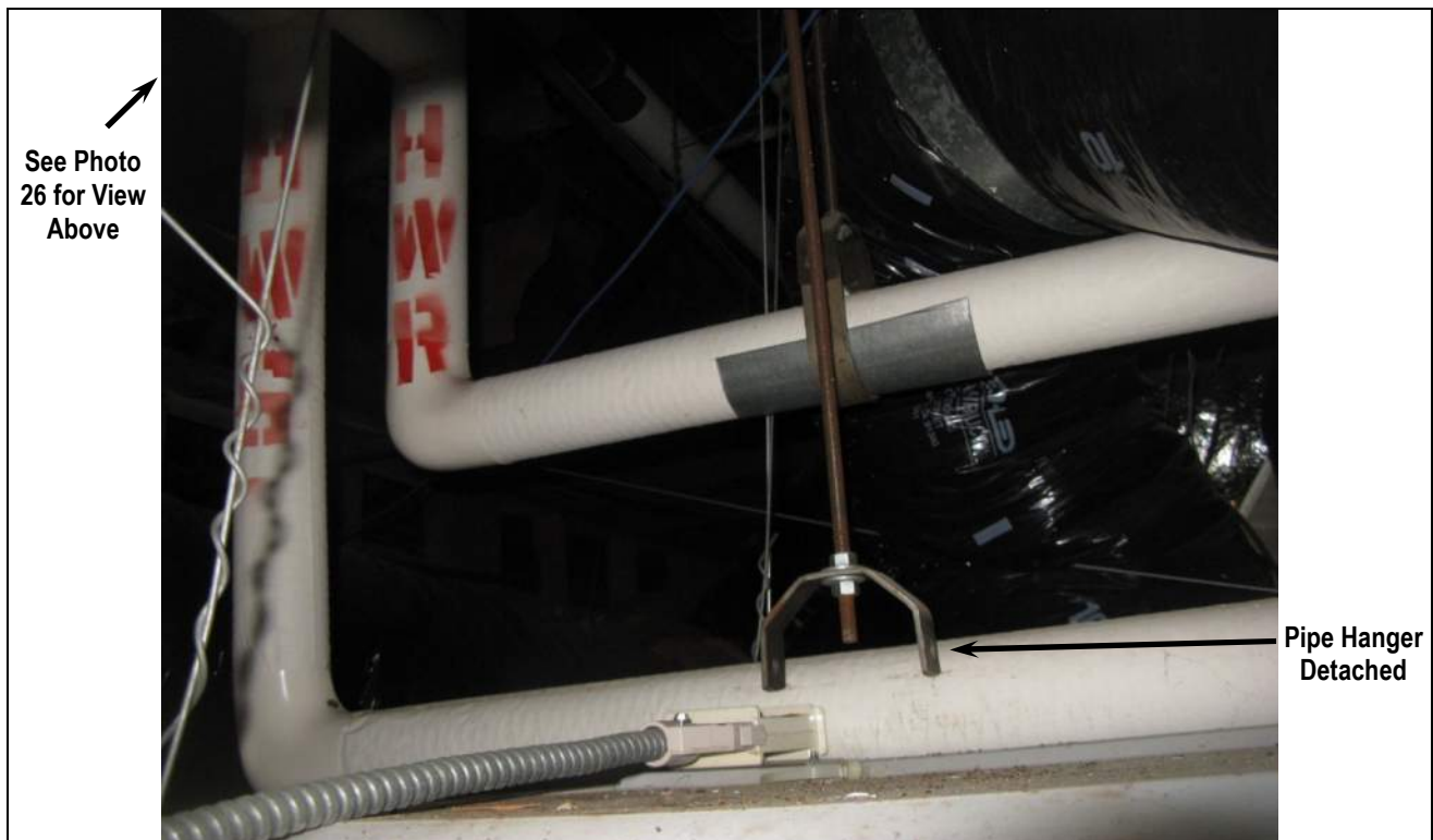
Photo 25: Piping in Ceiling Above Computer Room
