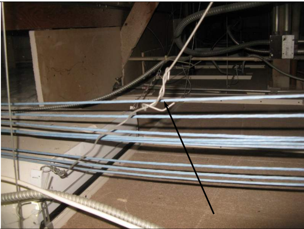
Photo 34: Improper Light Support Wire
