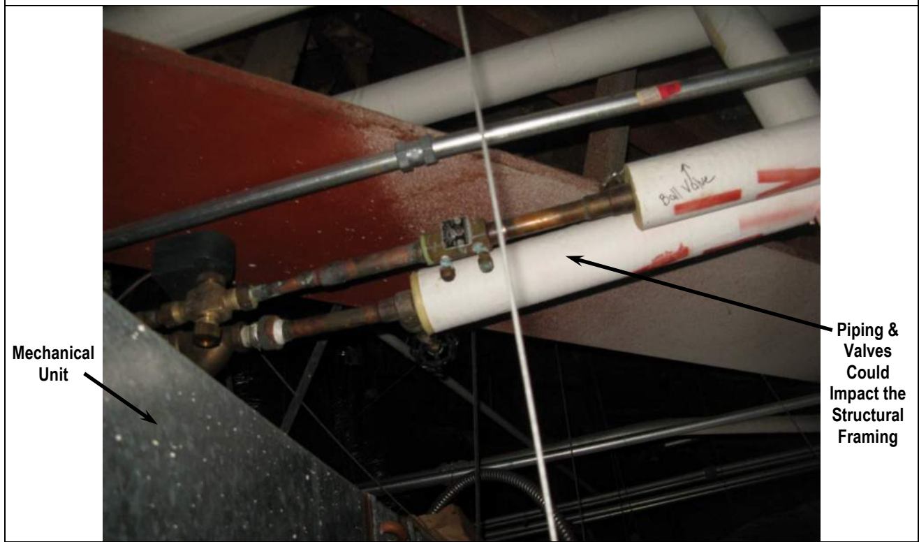
Photo 26: Water Piping in Ceiling Above Computer Room
