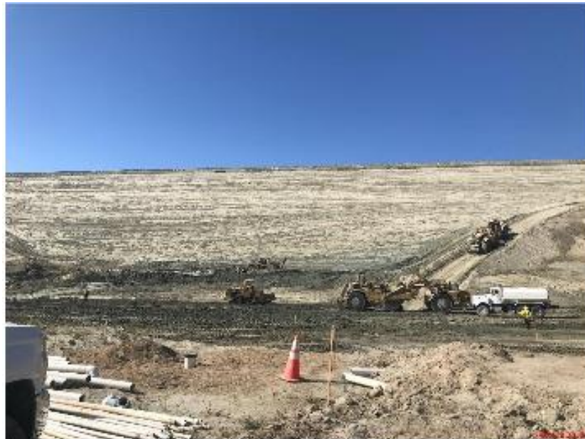
Main Dam Fill Operation at Elevation 412
