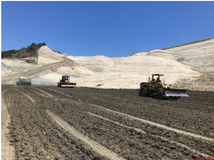
Compaction Work at Trampas Canyon Main Dam Embankment Butler June 2018 Construction Progress Report
