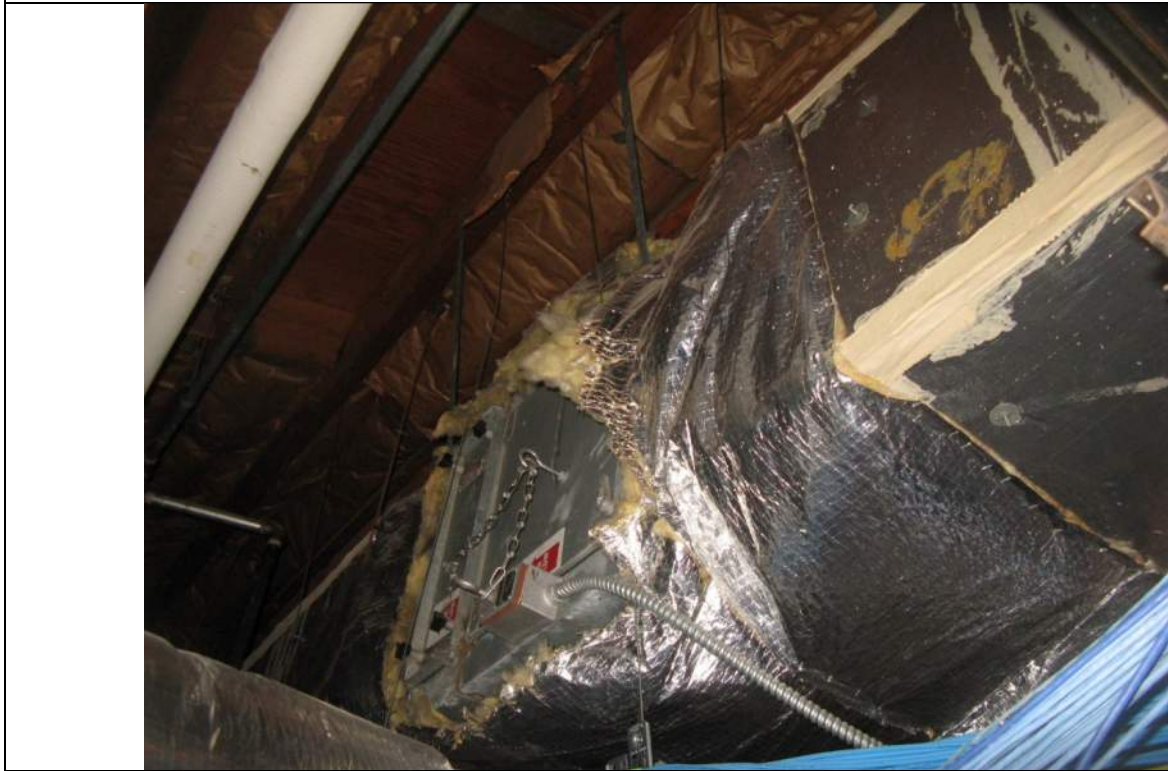
Photo 28: Typical In-Line Mechanical Unit without Seismic Bracing
