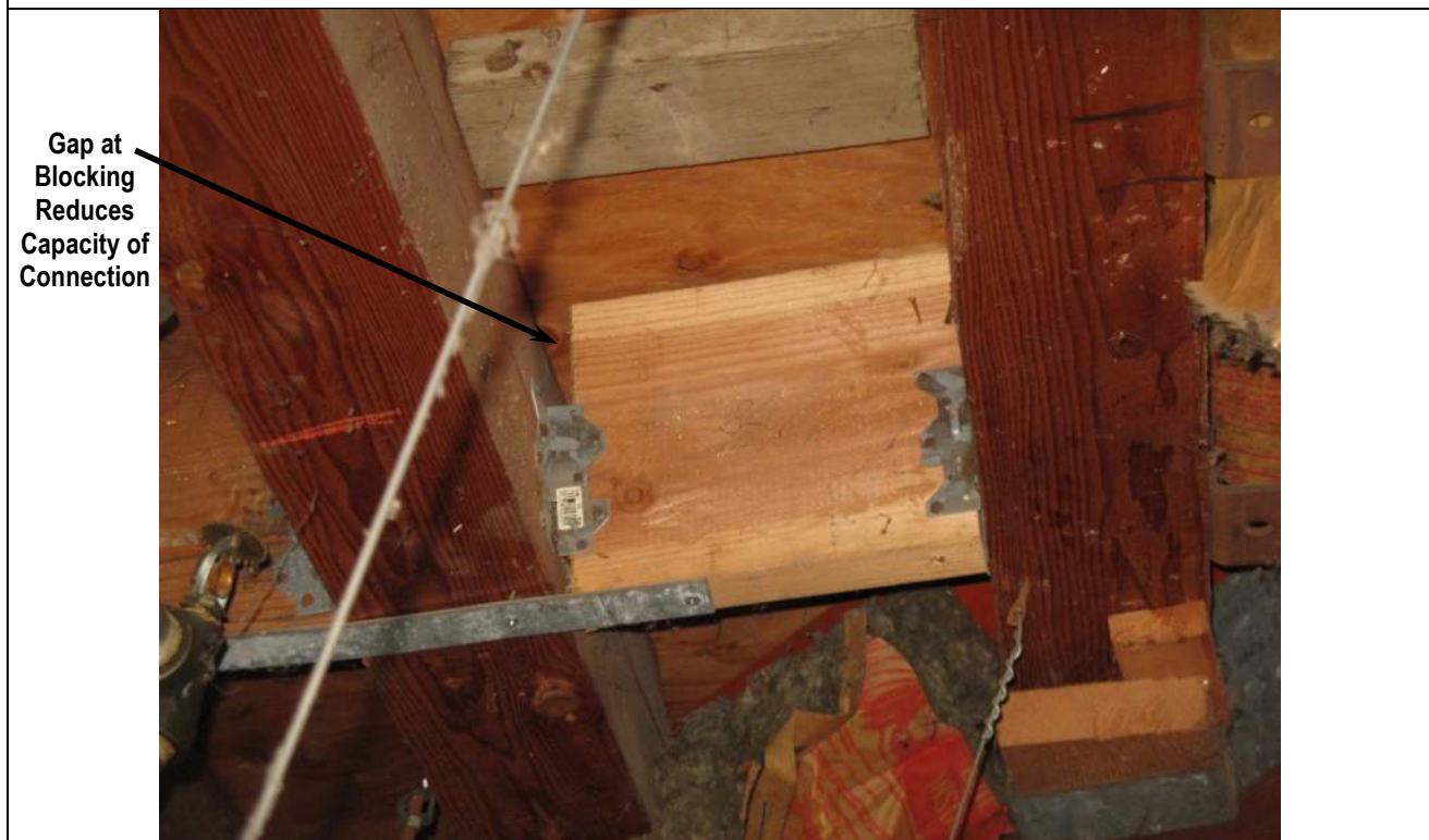
Photo 10: Close-up Showing Gap at Seismic Blocking
