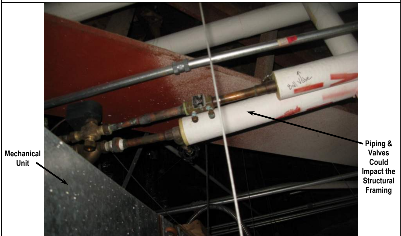
Photo 26: Water Piping in Ceiling Above Computer Room
