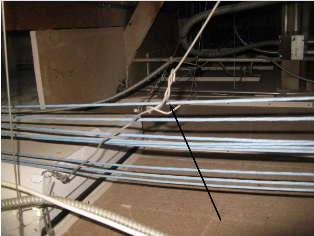
Photo 34: Improper Light Support Wire
