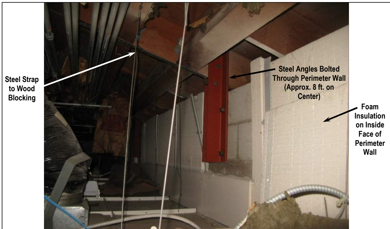
Photo 9: Typical Out of Plane Wall Anchorage Connection
