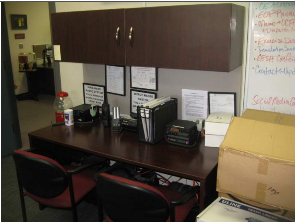
Photo 20: Unrestrained Communications Equipment
