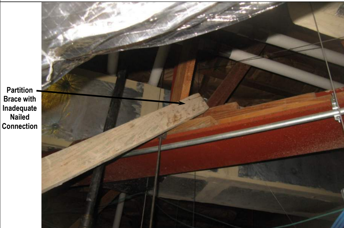
Photo 14: Interior Partition Bracing Connection
