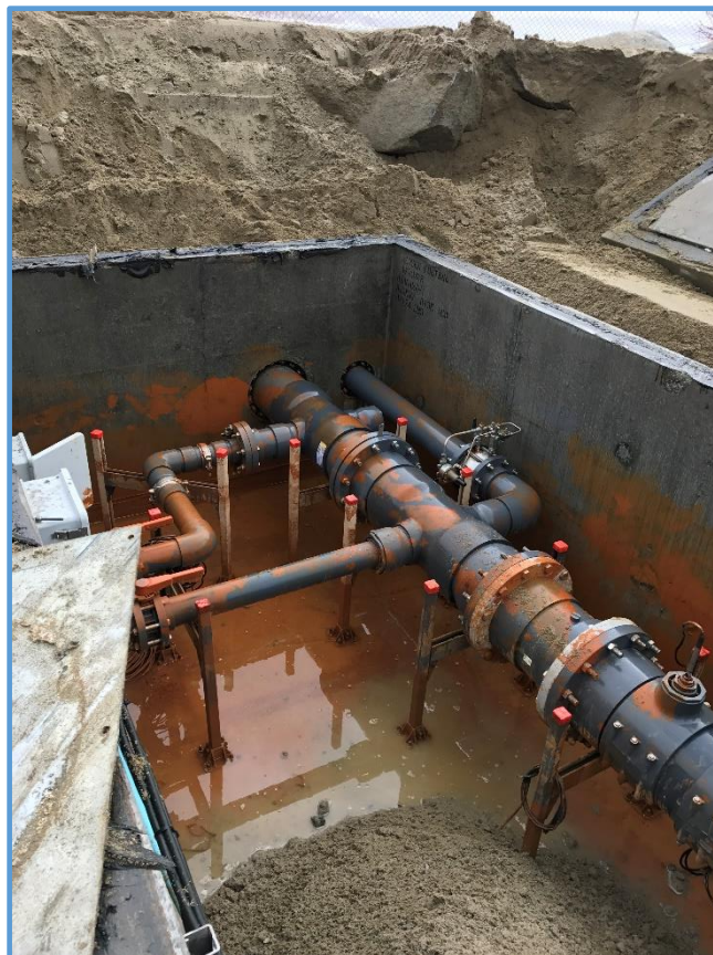
The valve vault on the beach at the wellhead
