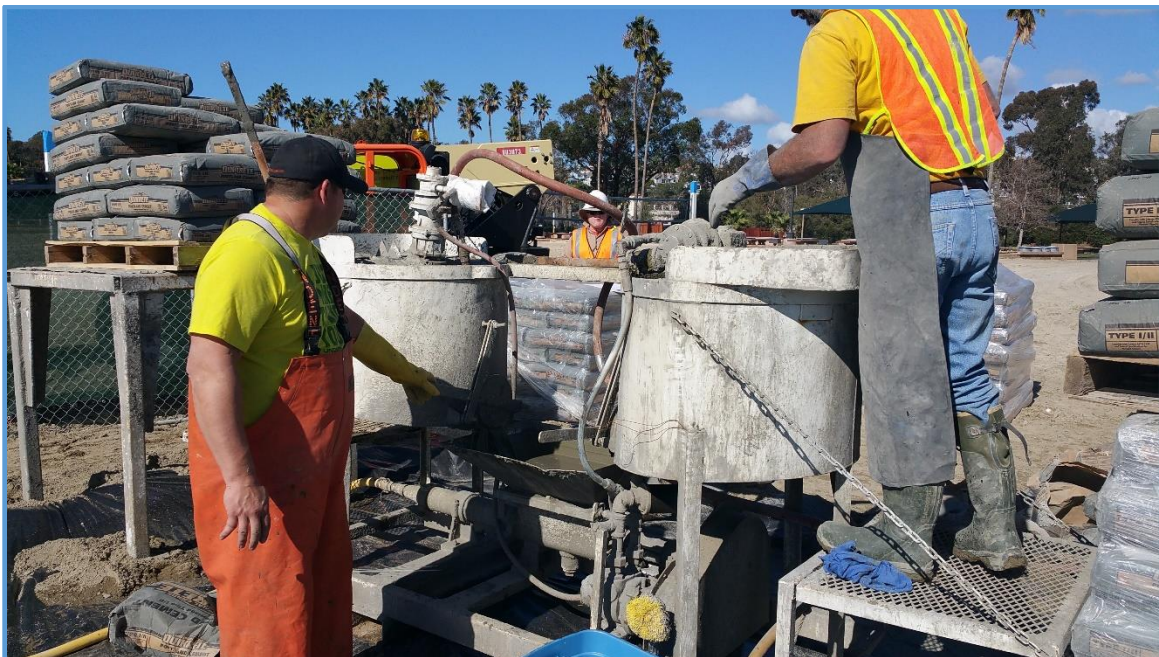
Mixing of grout for pumping into the abandoned well
