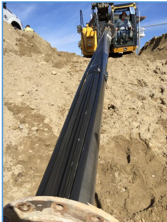
Cables and pump column being removed
