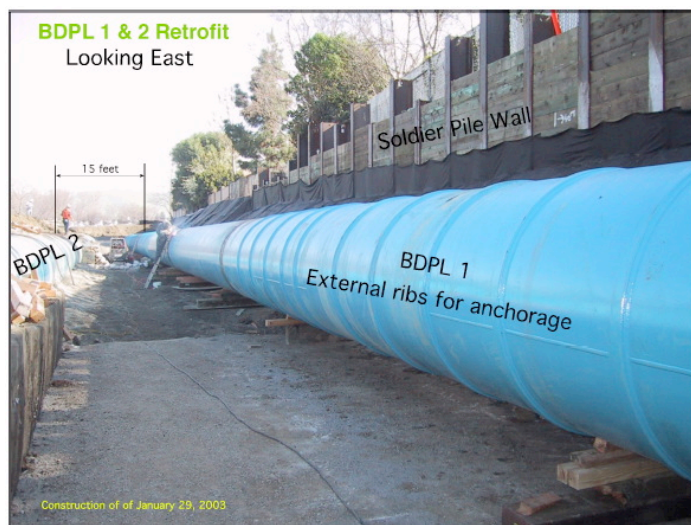
BDPL 1 and 2 Fault Crossing Design Details
