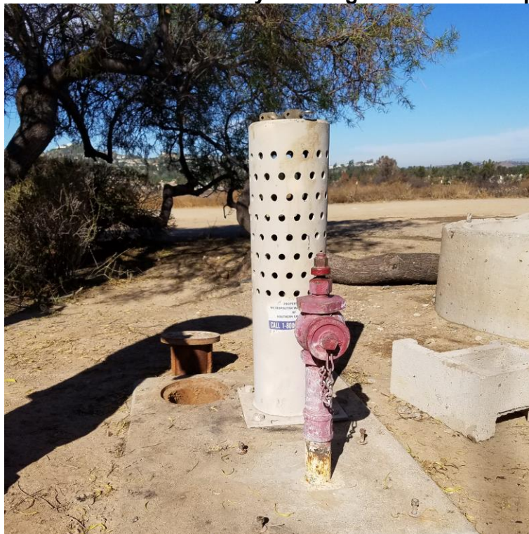
Small Connection Utilized by Fire Engine for Water Supply
