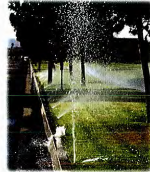
How often is this site checked? Reading a meter and comparing it to actual ET could help discover this problem before the water bill comes.
