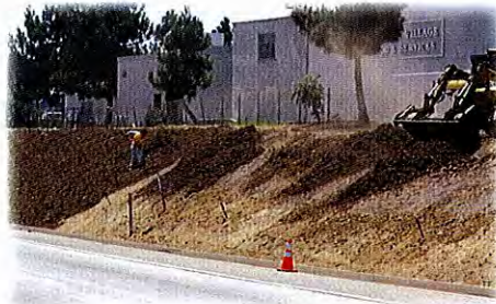
Mulch that is shredded does stay in place on hillsides. CalTrans shown mulching miles of freeway landscapes.
