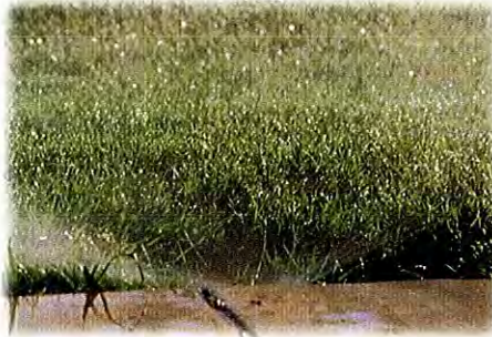
(Above) Pop-up spray head that does not reach above the grass. (Right) All heads were repaired or replaced with higher pop-ups. This retrofit costs less than over-watering.
