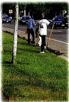
Raising irrigation heads to clear fast-growing turf
