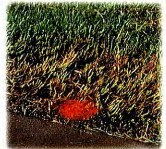
(Above) Pop-up spray head that does not reach above the grass. (Right) All heads were repaired or replaced with higher pop-ups. This retrofit costs less than over-watering.
