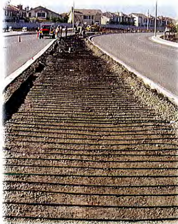
(Below) New streetscape with sub-surface irrigation. (Bottom and below, next page) Streetscape before; and after, with 50 percent less water and reduced paving damages.
